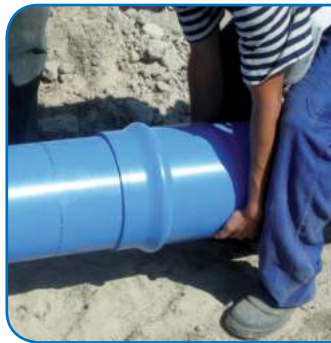
Align the pipe and place the spigot end inside the socket or bell.
