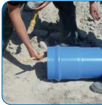
Apply lubricant on the chamfer of the spigot end and in the rubber ring joint.
