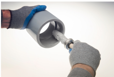
Apply cement to ID of pipe
