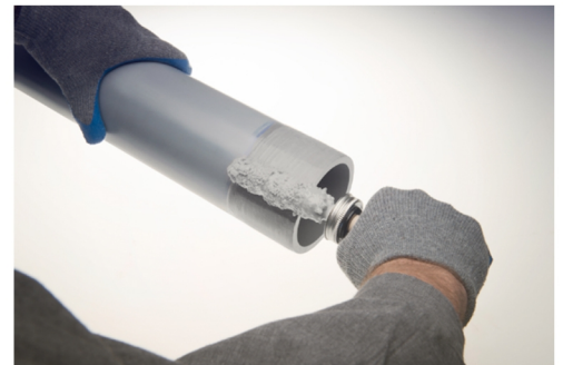
Apply cement to OD of pipe
