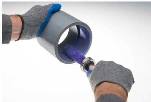
Apply primer to ID of fitting
